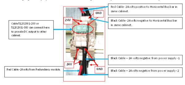
The following figure displays the terminal block wiring for COTS power Meanwell non-redundant system.
