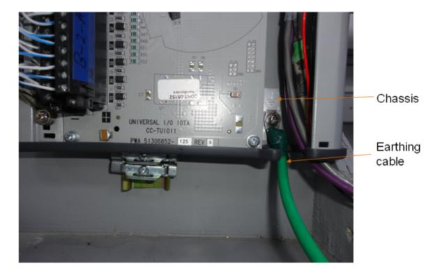
Figure 164: Grounding connections
